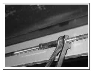
Thread a 1/2" jam nut onto the 1/2" x 126" rod. Then, thread the 1/2" x 126"Rod into the 1/2" coupler. This can Be started by hand from underneath, and adjusted and tightened from the flange end using a 1" open end wrench.
